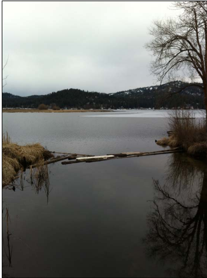
Figure 4: Looking west toward the lake from the outlet gate structure on March 5, 2013.
